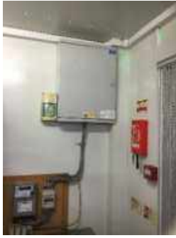
Electric isolation and meter, kitchen pod, dedicated supply, not on older plans
